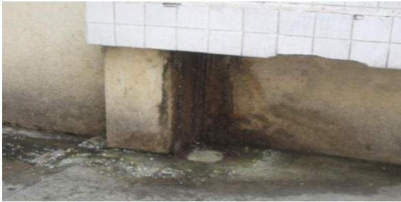
Plate 10: Poor Drainage system in Zeenat Mahal, Kamla Market
