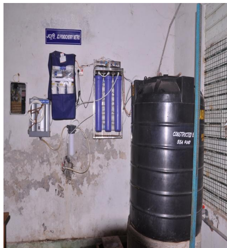
Figure -9 Installation of RO system for safe drinking water
