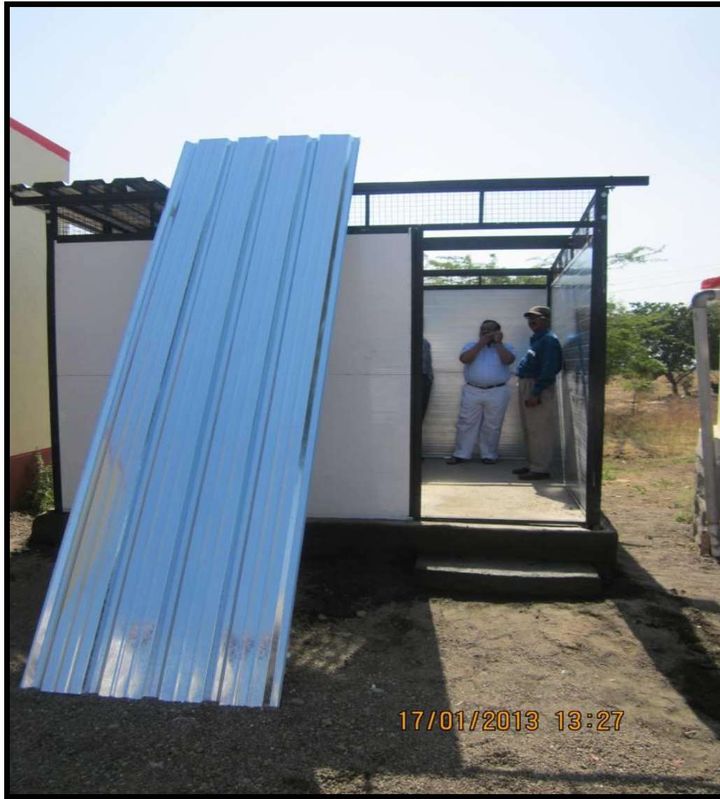
Erection Work In Progress
