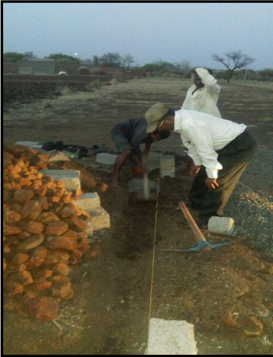
Plinth Construction In Progress
