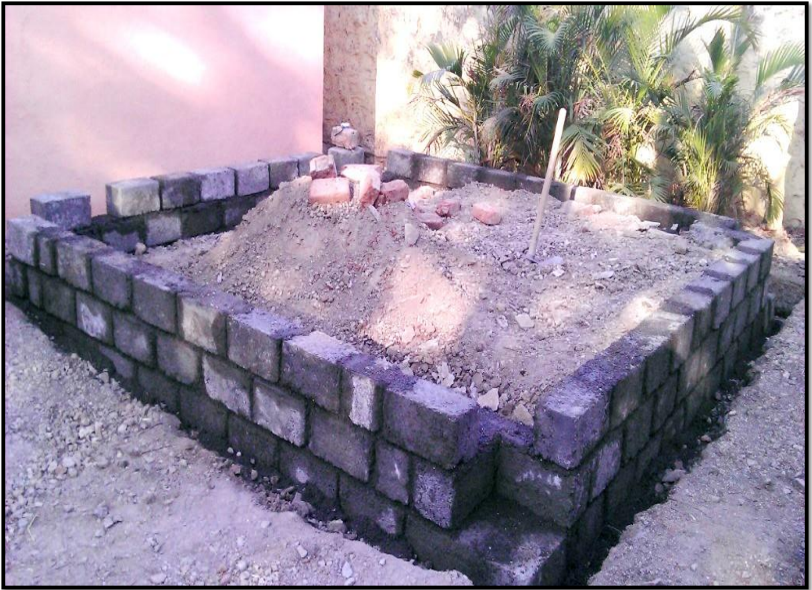
Plinth Construction In Progress
