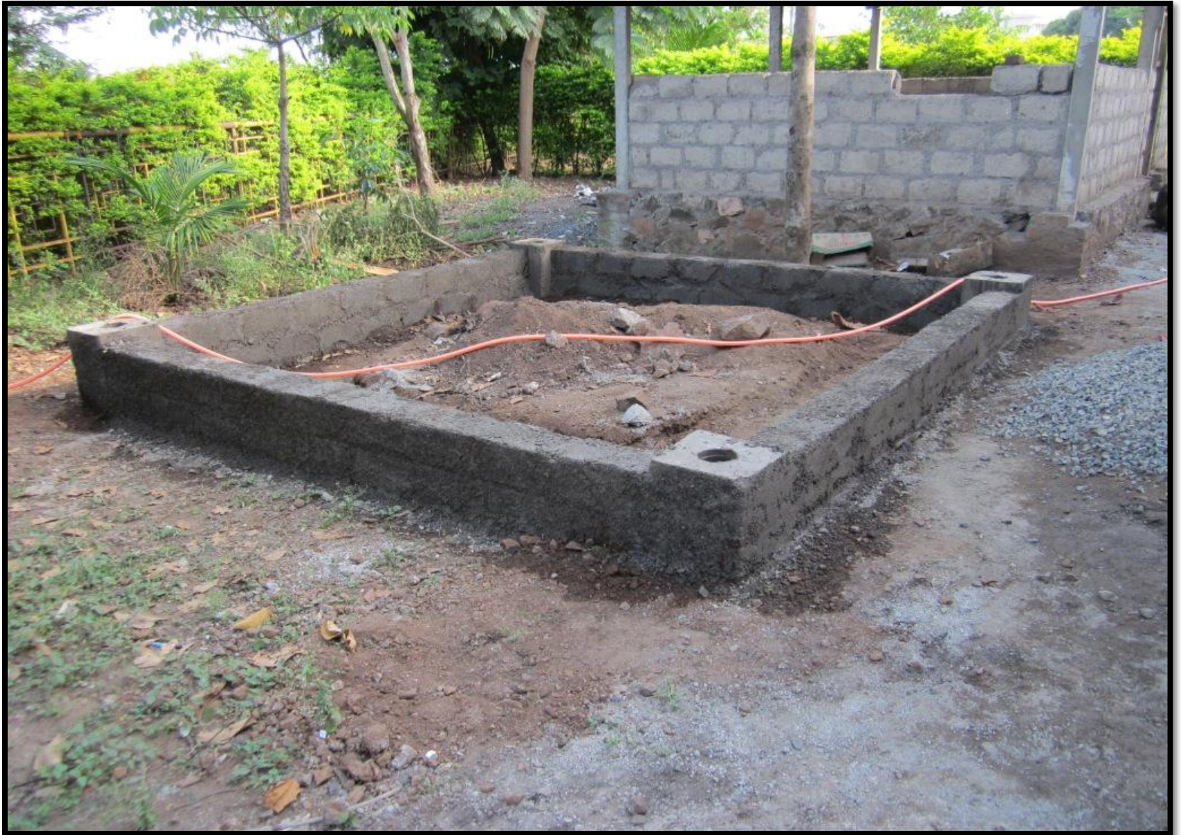
Plinth Construction In Progress
