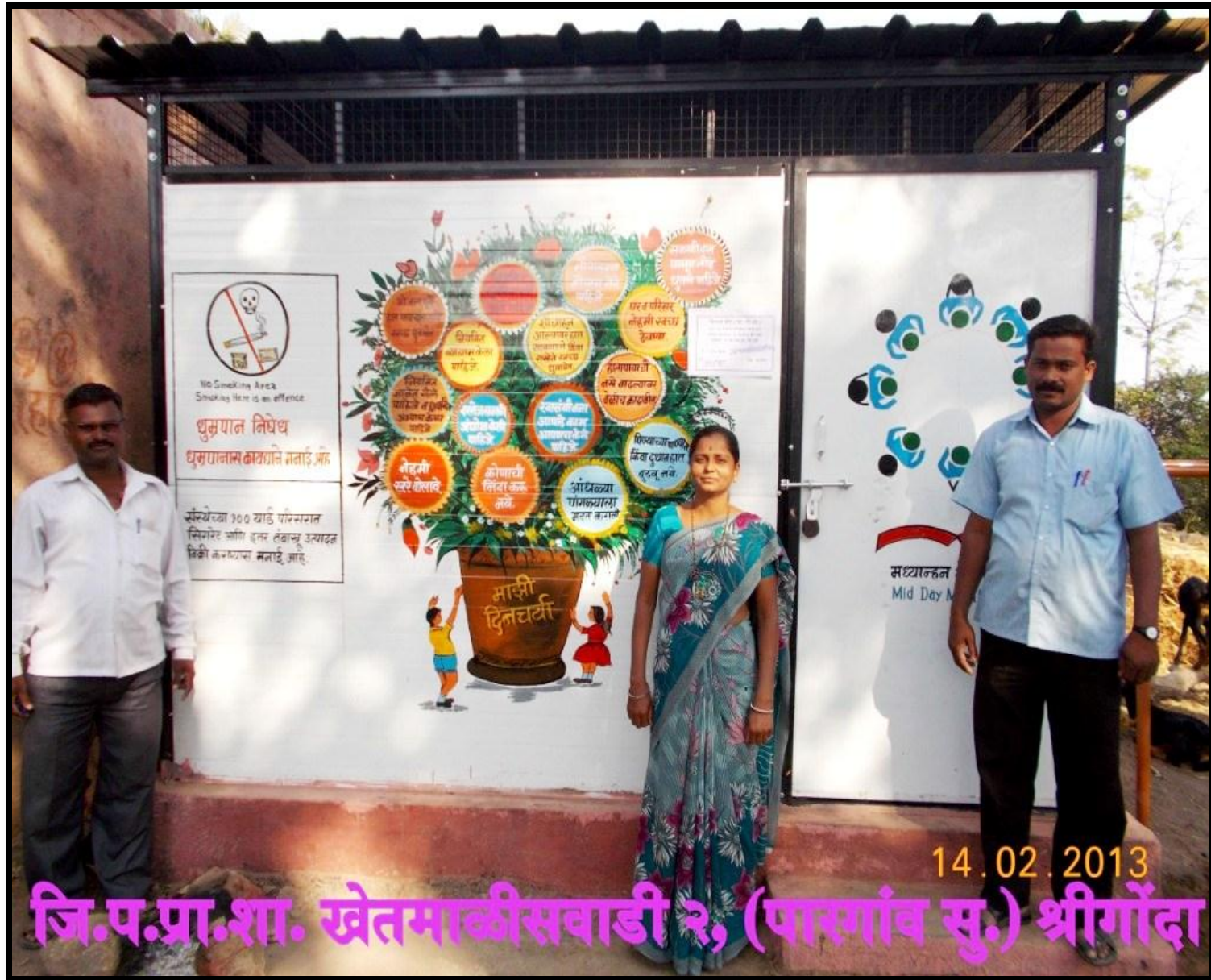
Handing Over of Completed Kitchen Shed
