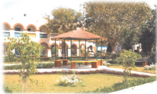
Fig. 3.6 : A shed made from waste material in a school
