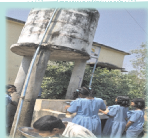
Fig. 3.13 : Tanks for storage of water
