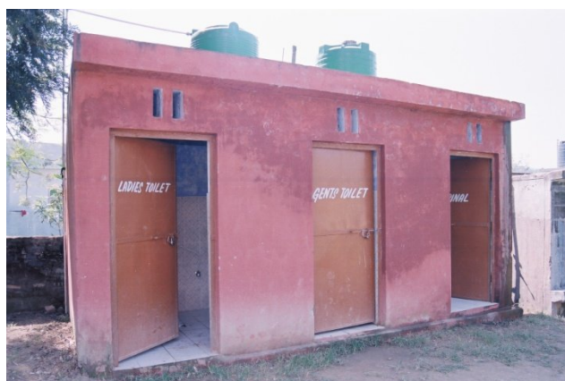
Toilet at GHS Garhi, Udhampur
