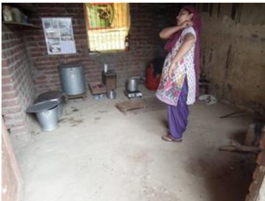
POORLY CONSTRUCTED KITCHEN SHED IN GPS, ROSHAN WALA
