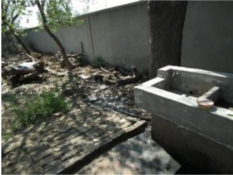
POOR SANITATION OF WASHING AREA IN A SCHOOL
