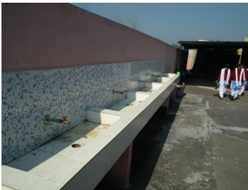
WELL CONSTRUCTED DISH WASHING AREA IN A SCHOOL (GSSS, Kalitran)
