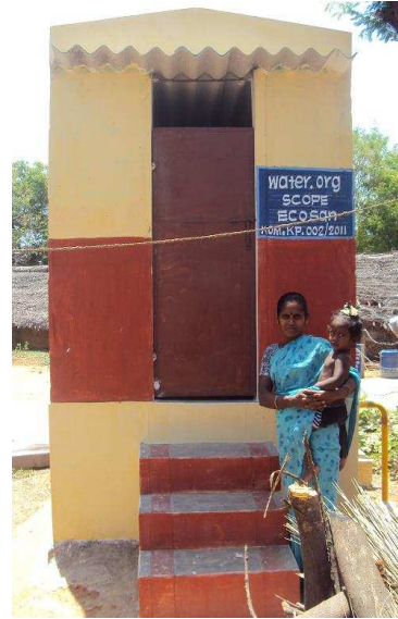
Ecosan toilet superstructure with brick, cement, and RCC roof and iron door
