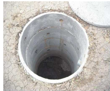
Fig 4.2 Single pit toilet with provision of a second pit Fig 4.3An open ring channel pit
