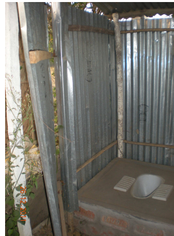
Superstructure with G.I. sheet
