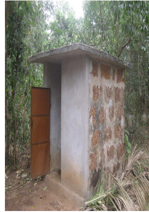
Superstructure with stone wall, RCC roof and iron door
