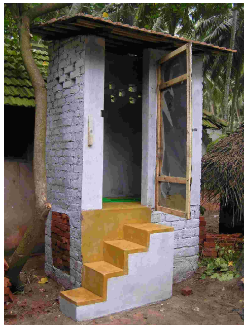
Ecosan toilet superstructure with brick, cement, and red stone roof and Tin door
